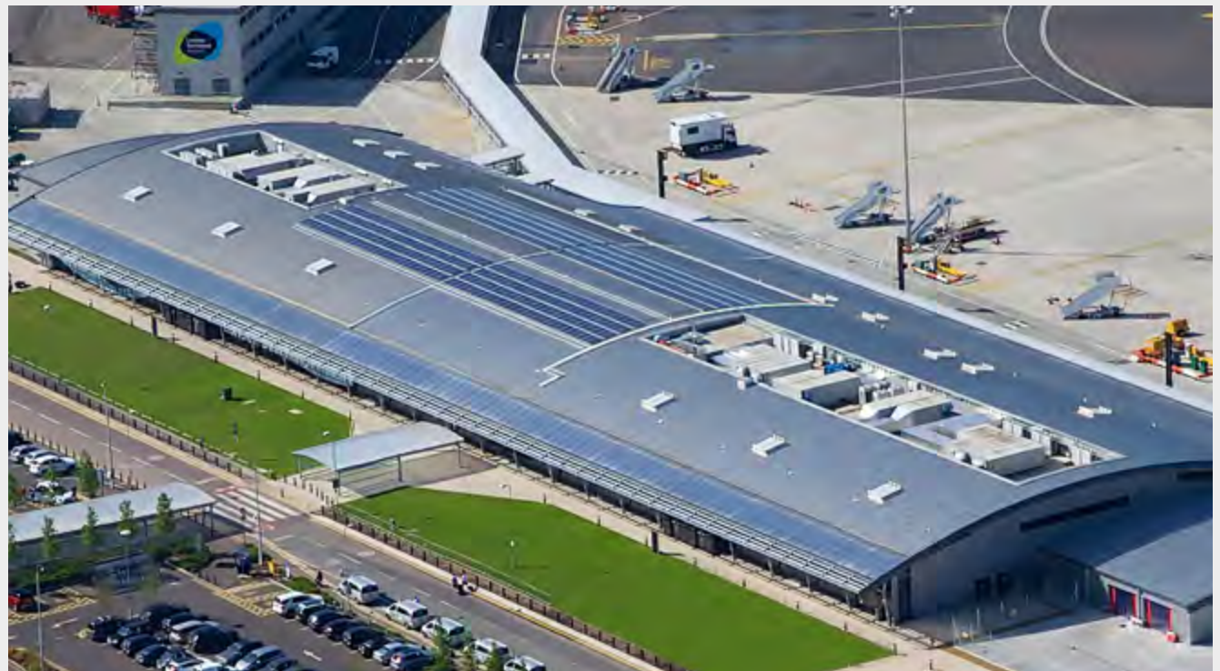
Solar panels installed on the roof of the new terminal.
